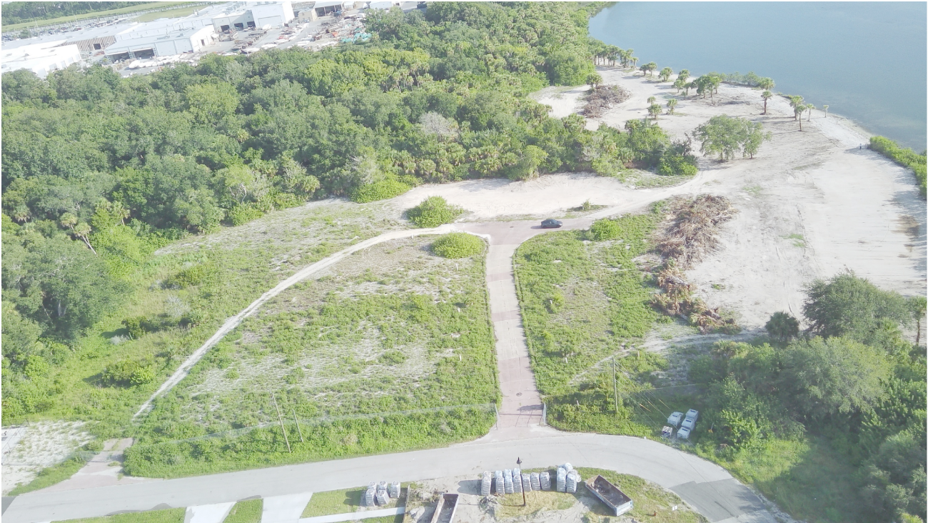
EXISTING SITE FACING NORTH
