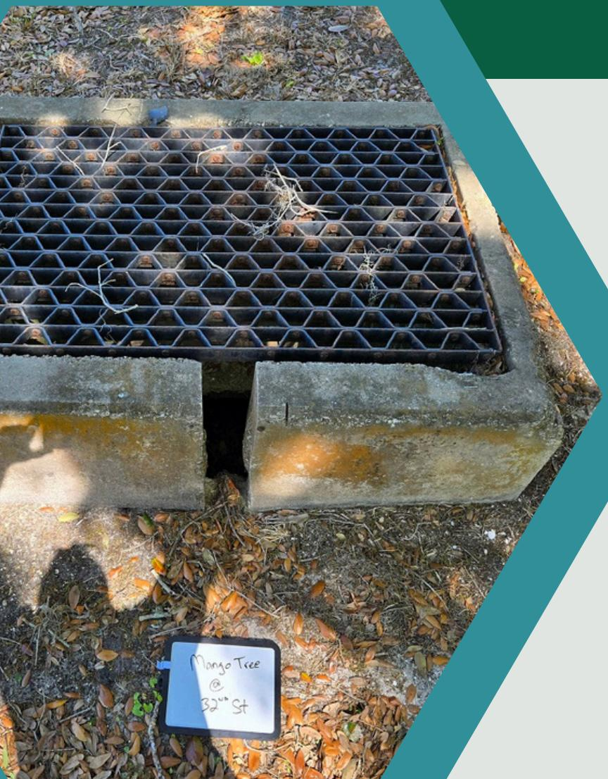
In response to urgent flooding concerns in past years, City staff intentionally modified 40 drainage basin boxes as a temporary measure to move water more quickly during heavy rain events. While this provided short-term relief for neighborhoods, it also altered the basins from their original engineered design. Over time, these changes required formal restoration to ensure the system remained in compliance with regulatory standards and could function properly for the long term.
