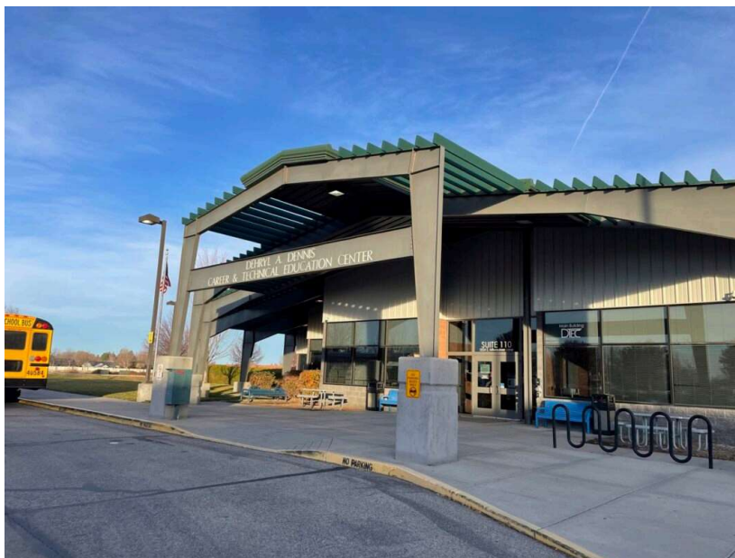
The main building at Boise School District's Dennis Technical Education Center off of Victory Road. Photo: Margaret Carmel/BoiseDev
